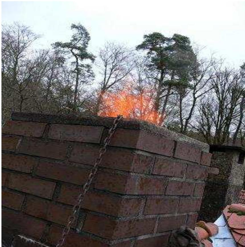
Fig 4 Picture from the process of burning out the chimney flue
