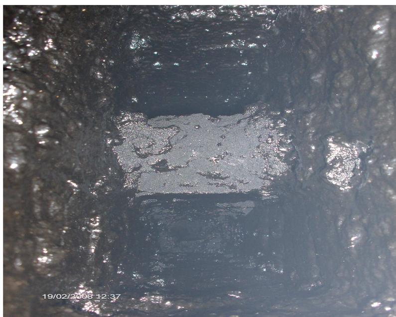
Fig. 1 Glassy soot in the chimney flue
