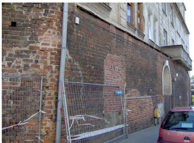
Rys. 1 Widok ogólny muru obronnego [2] Fig. 1 General view of the wall [2]
