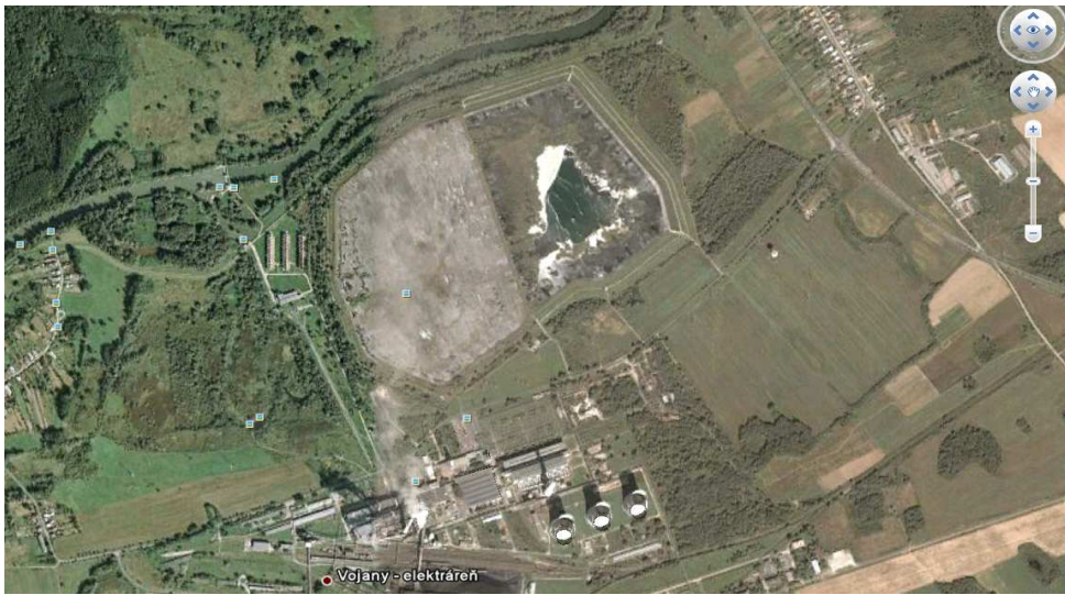
Fig. 4 Plain desludging site of ash waste
