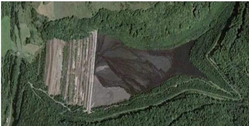
Fig. 2 Valley desludging site for metalliferous waste
