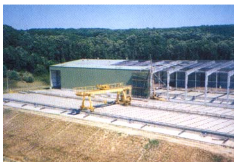
Fig. 2 Building of the temporary overlap of 1st double-line of storage boxes
